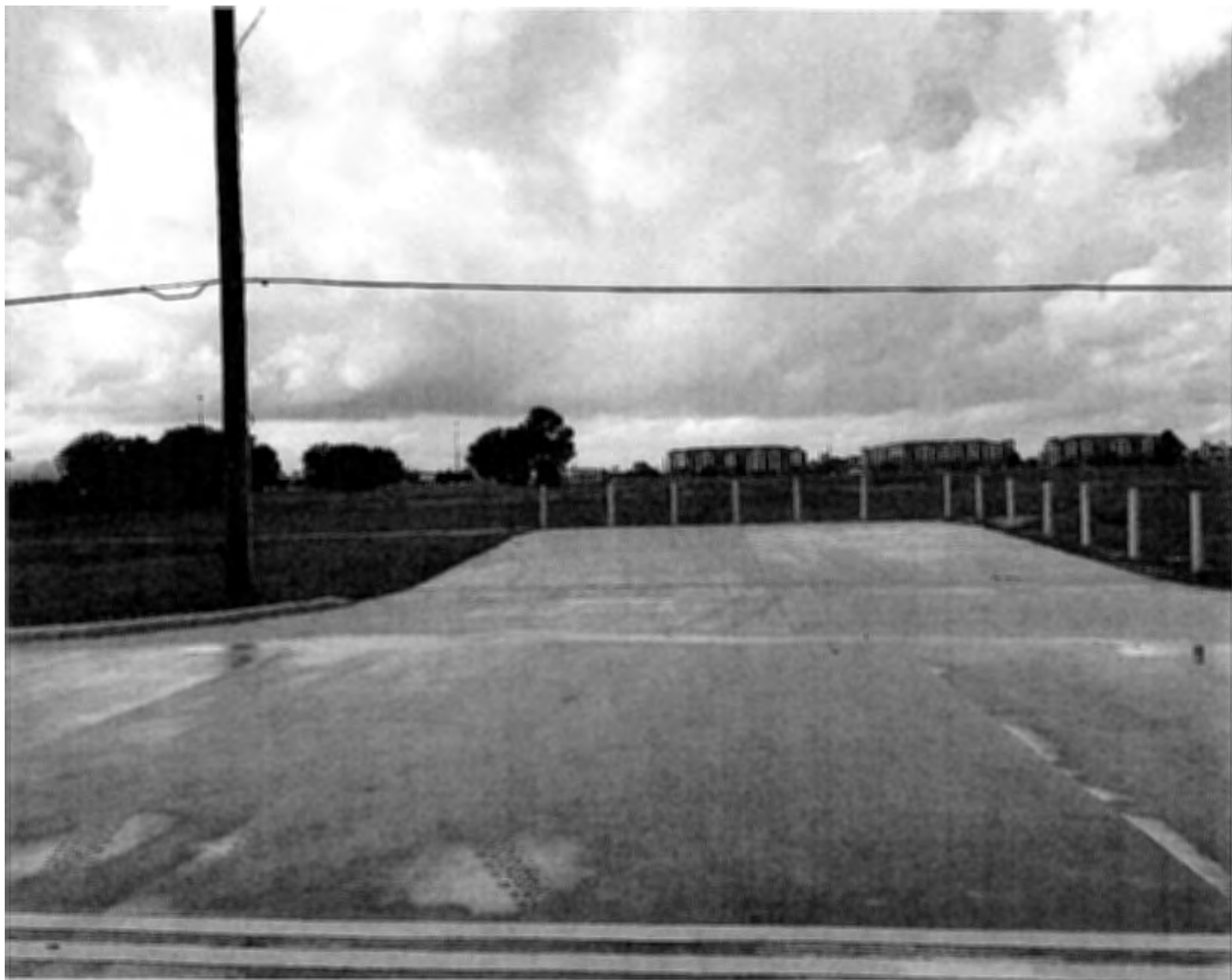
Newly constructed driveway north of site
