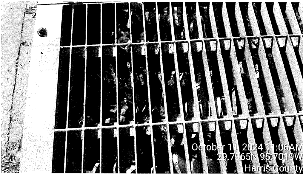
Trash Under Bar Screens - Ponds B
